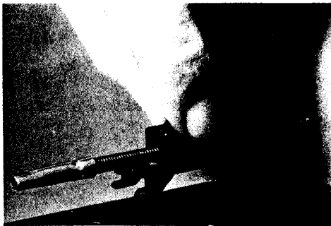
Figure 2.5. Installation of mounting bracket.
