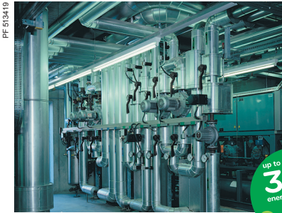
ATV12 controlling a pumping station
